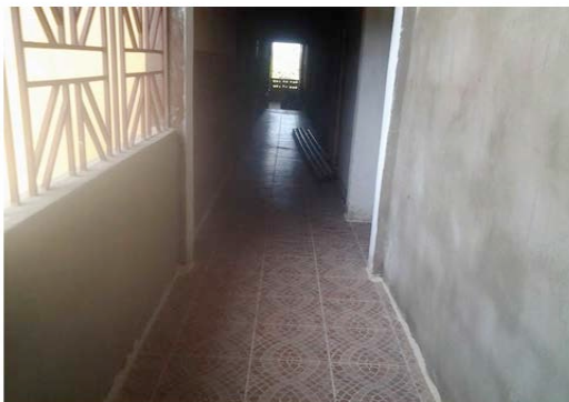
Hallway interior of Isolation Ward
